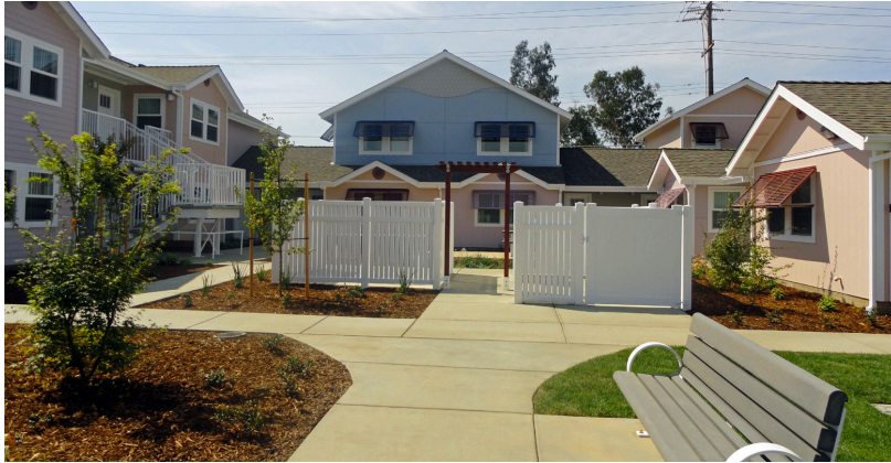
Photo credit: Sunseri Construction
