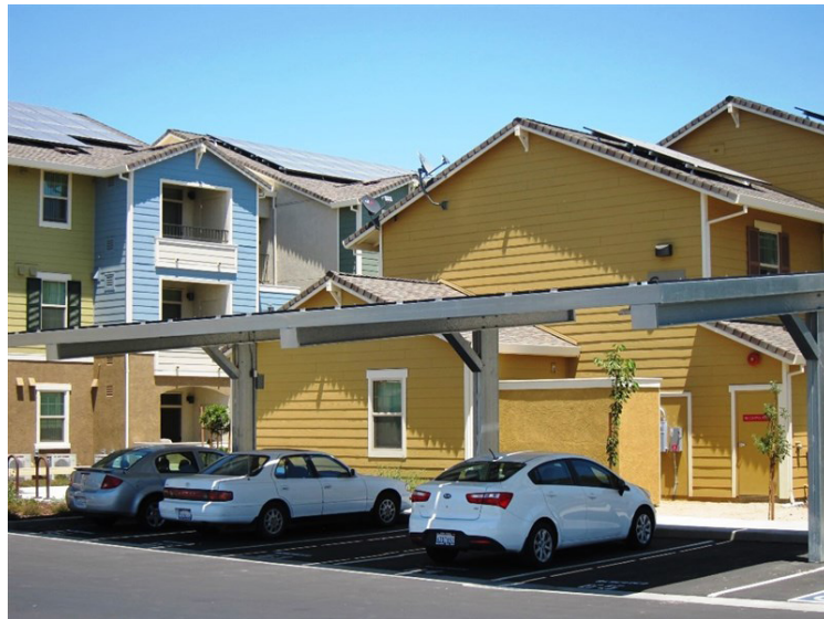
Solar panels built on structures above parking spaces feed the electric grid. Photo courtesy Amy Quinton / Capital Public Radio
