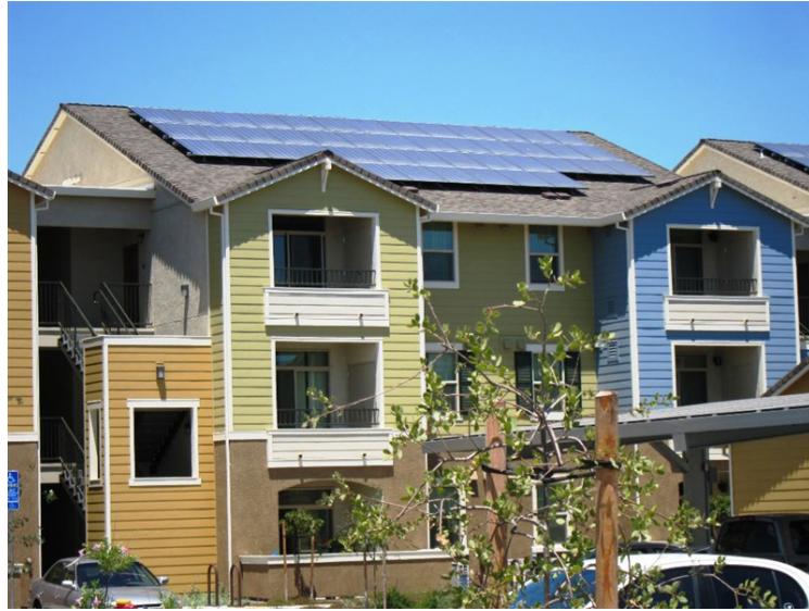
Solar panels adorn south-facing rooftops also provide electricity for the units. Photo courtesy Amy Quinton / Capital Public Radio
