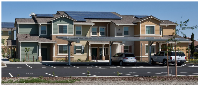
The development at Spring Lake is the first multifamily rental community to be certified under the DOE Zero Energy Ready Home program.
