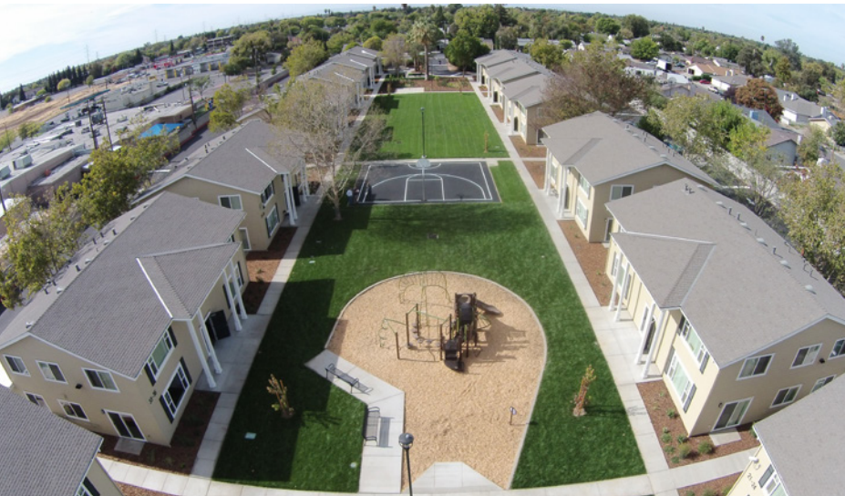
Shown here is an aerial photo of one of the three Sacramento communities at Mutual Housing.
