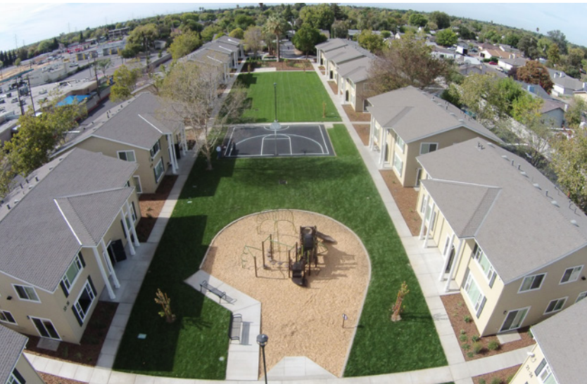
Shown here is an aerial photo of one of the three Sacramento communities at Mutual Housing.
