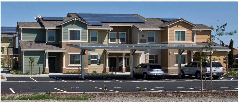
The development at Spring Lake is the first multifamily rental community to be certified under the DOE Zero Energy Ready Home program.
