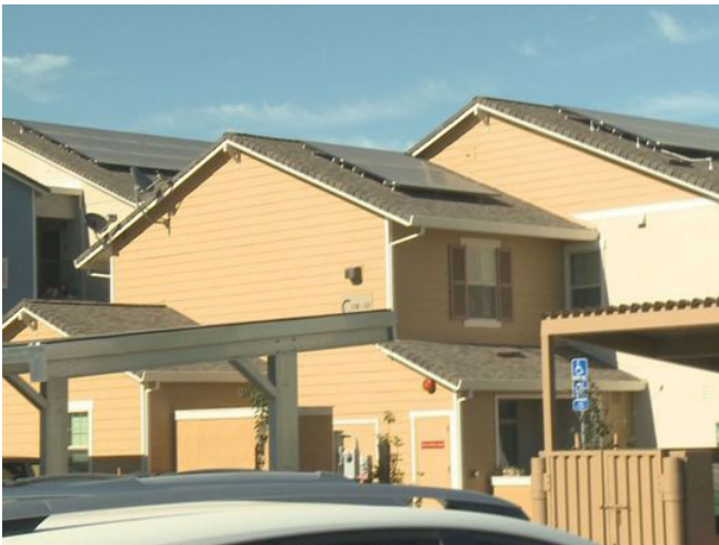
The apartments buildings at the Mutual Housing at Spring Lake complex all have solar panels on the roofs, driving energy costs down for renters. (Photo: Lee Maxwell/News10)
