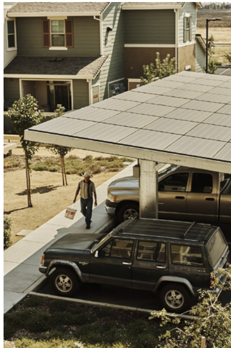
Even the carports at Mutual Housing at Spring Lake are covered with solar panels. Photo courtesy Cait Oppermann
