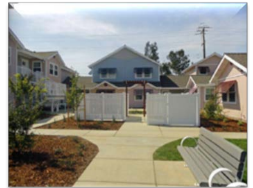
Highlands, a multi-family development operated by Sacramento|Yolo Mutual Housing Association, received 121 points from Oakland-based Build It Green (BIG).
