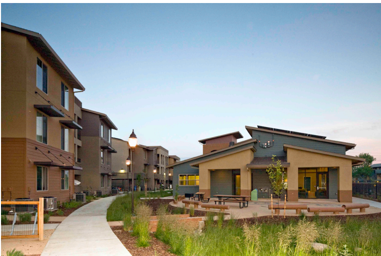
Green building practices help residents of New Harmony Mutual Housing on Cowell Boulevard in South Davis save money on their energy bills.
