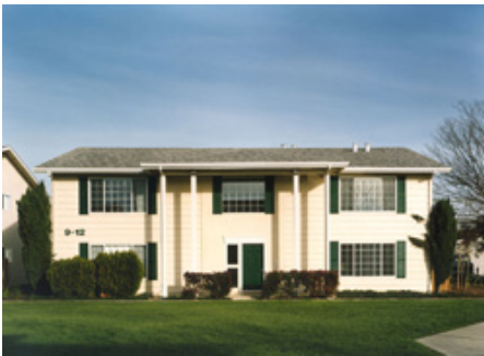
Greenway Mutual Housing received funding to be rehabilitated. Photo courtesy of Mutual Housing California.
