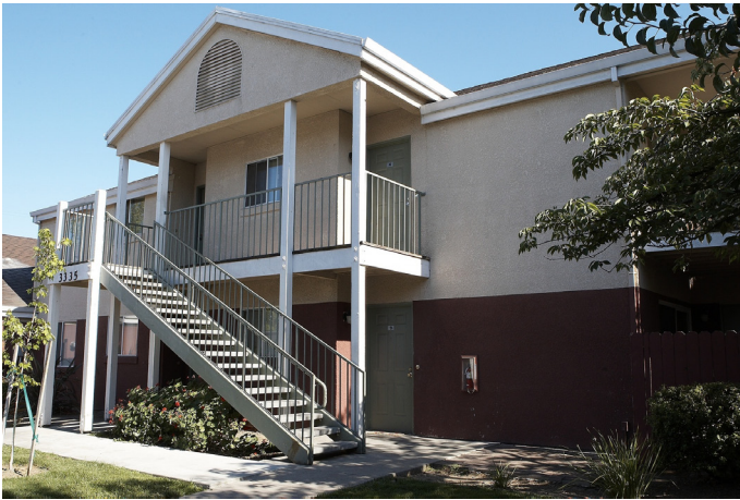
Mutual Housing California received the county's first BIG rehab rating for the rehabilitation of Norwood Mutual Housing. Photo by Roy Wilcox.
