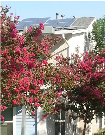
Moore Village Mutual Housing Community now has solar panels.
