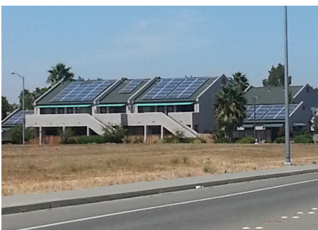
Solar panels at Twin Pines Mutual Housing Community will help residents with utility costs.
