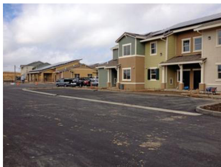
Homes are starting to take shape at the new Mutual Housing community at Spring Lake. Courtesy of Vanessa Guerra.
